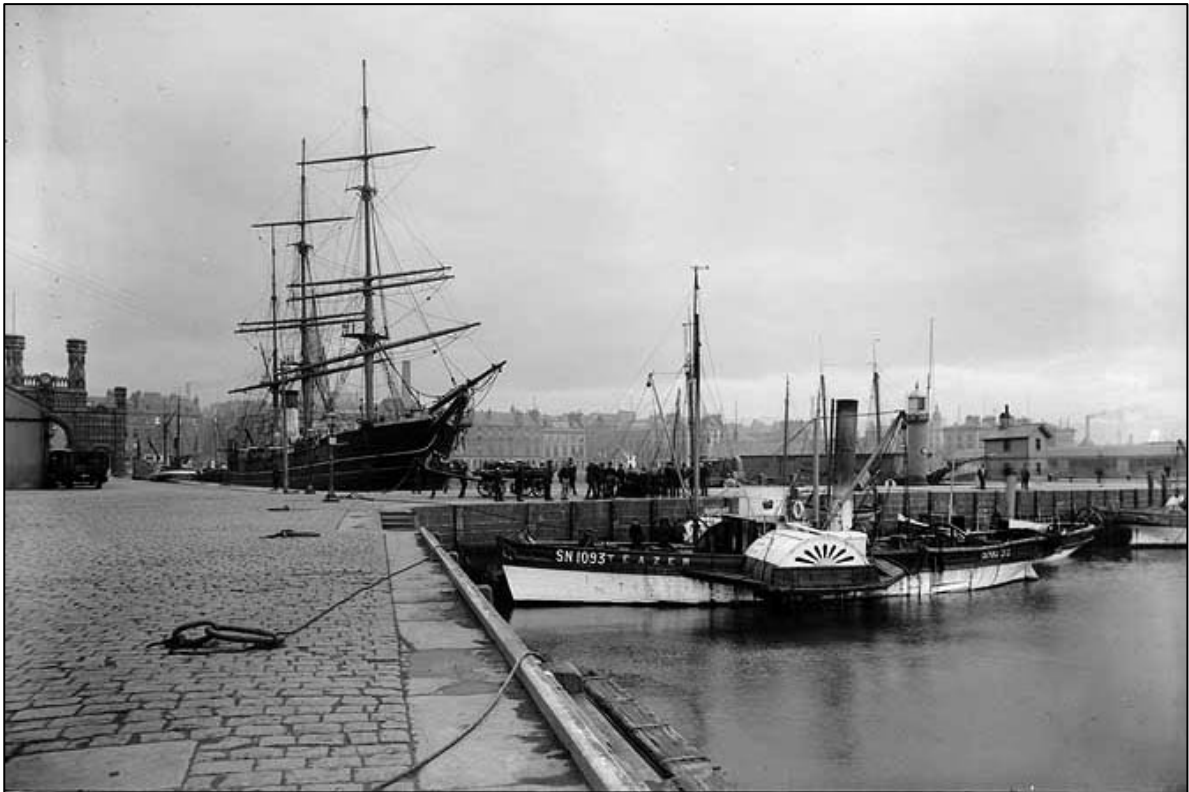
Figure 8a: View of Dundee Docks, showing in situ Timber Buffering (Wilson, 1895a)
