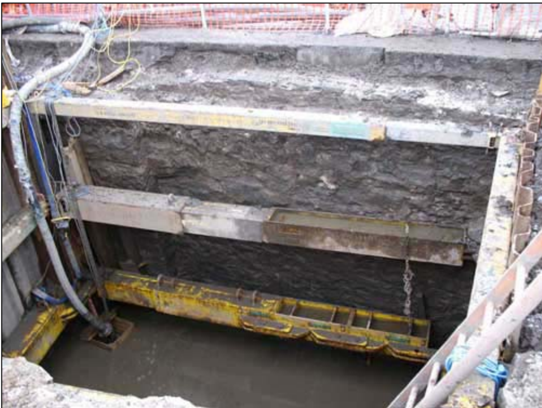
Figure 5b: Inner Face of Inner Harbour Wall, Buttress to Left
